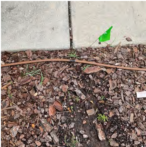
Zone #4 (Broken Drip or Micro Spray) - 06-01-26
