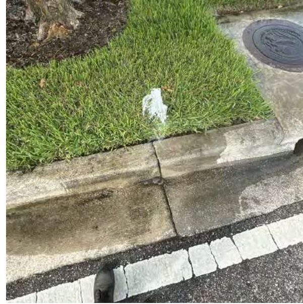
Zone #22 (Broken Head) - 06-04-26 9:17 am CDT
