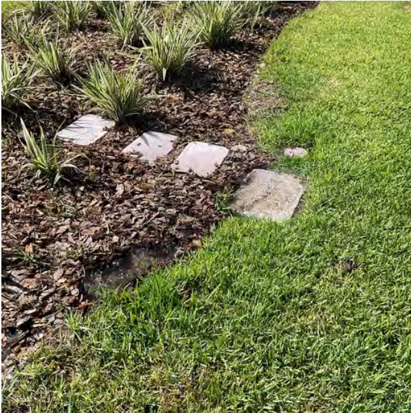
Zone #2 (Broken Lateral) - 06-09-26 5:39 am CDT
